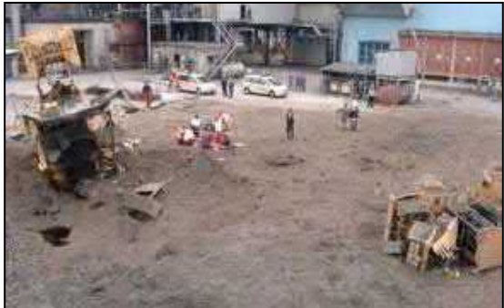
Destroyed piling rig and dump truck after detonation of WWII UXB in Austria – 2006.
